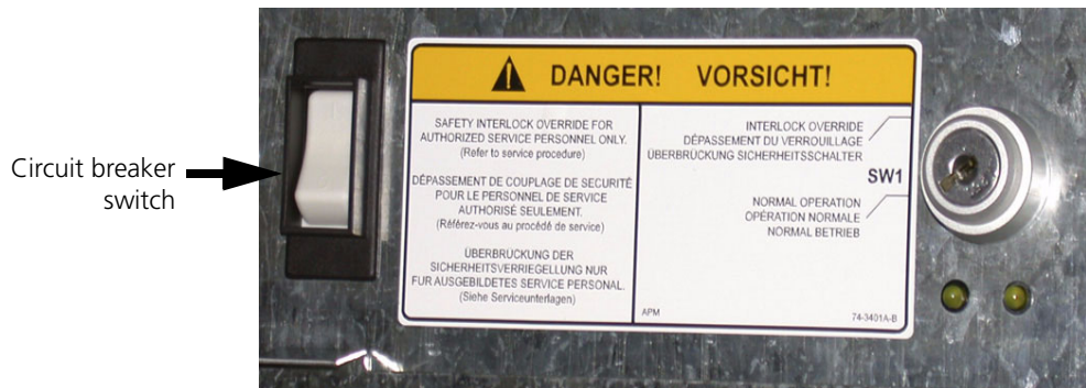
Figure 32: Circuit breaker switch
